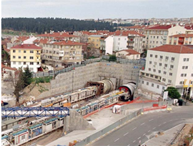
Fig. 5-2 Excavation in an urban area
