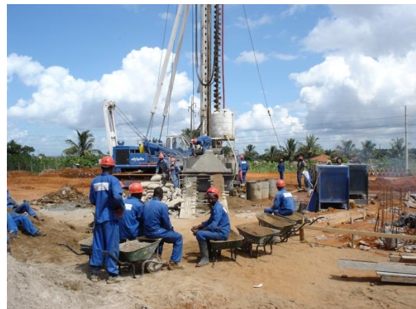
Figures 4 & 5 - Mechanised vs. labour intensive piling
