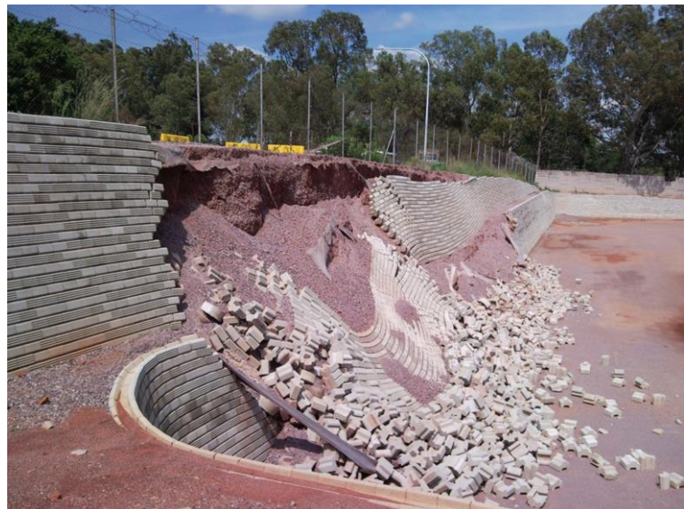
Figure 6 - Collapsed retaining wall
