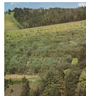
Figure 10. Soil-Bioengineering and its “Father” M. Schiechl (1922 - 2002), Austria. Examples of living soil reinforcement for highway embankments up to 60 m height (1963).
