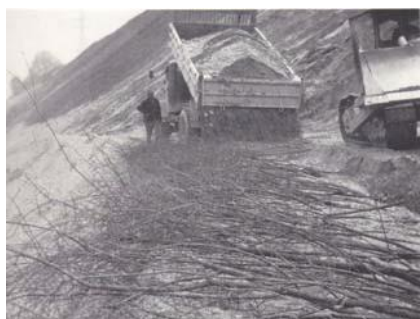
Figure 10. Soil-Bioengineering and its “Father” M. Schiechl (1922 - 2002), Austria. Examples of living soil reinforcement for highway embankments up to 60 m height (1963).
