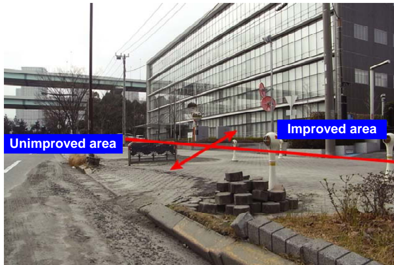
Photo 9 Successful ground improvement in the Tatsumi area in a man-made island of Tokyo
