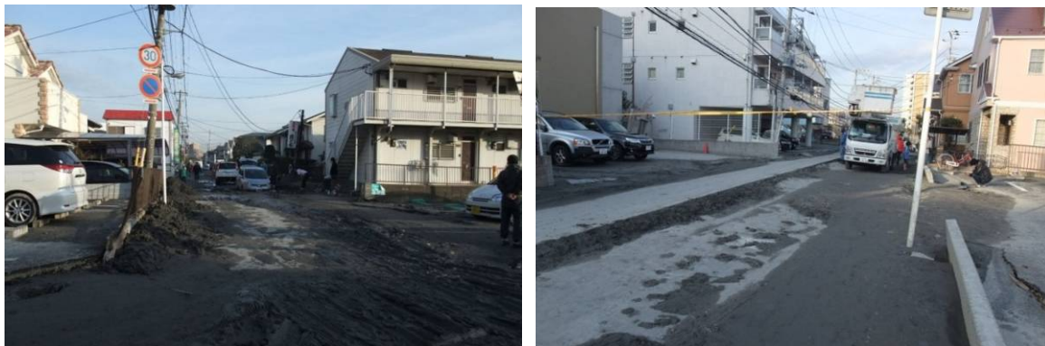
Photo 2 Damage in Urayasu City the next day
