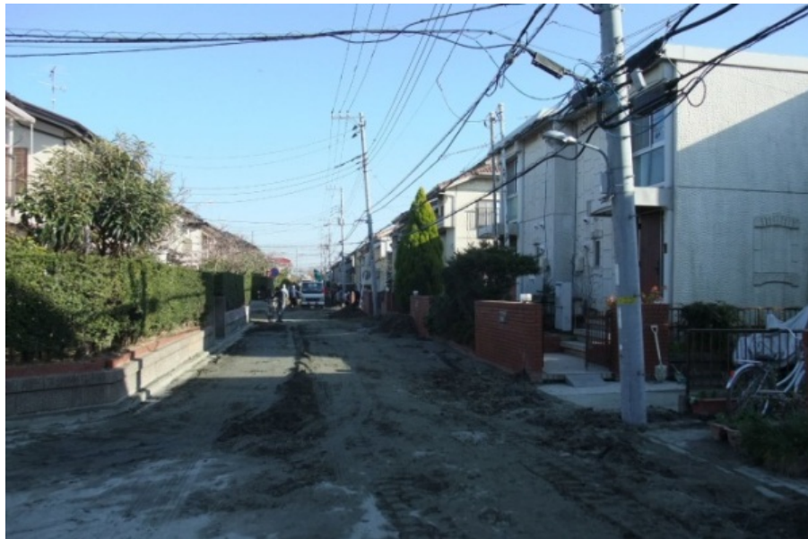
Photo 3 Damage in Chiba City on the third day after the earthquake
