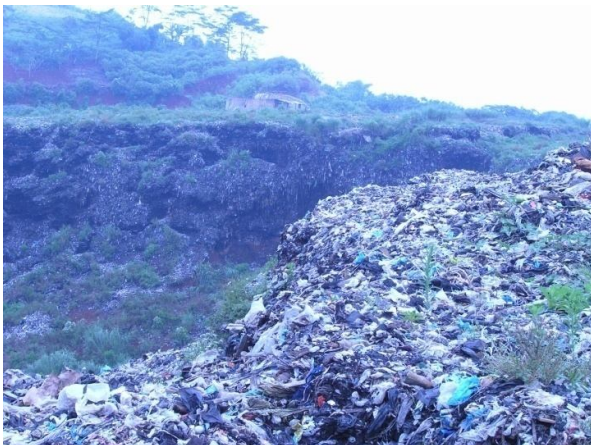
Photo 1 Top scarp of failed landfill
