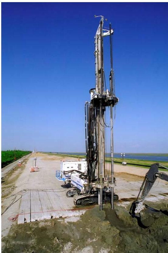
Figure 7. TREVIICOS Rig (Soilmec SR-90 - double shaft)
