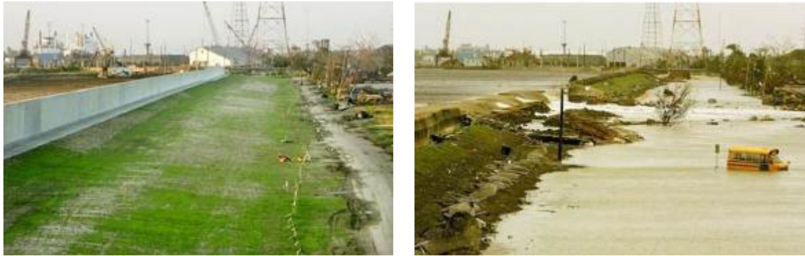
Figure 2 Damaged Section of Levee after Hurricane Katrina
