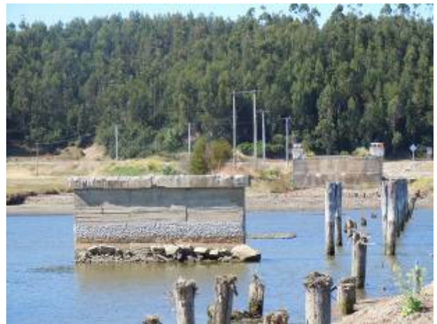
Subsidence of Tubul Bridge pier by 1 to 1.5 m because of subsoil liquefaction
