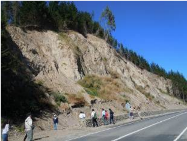
Failure of coastal slope near Concepcion
