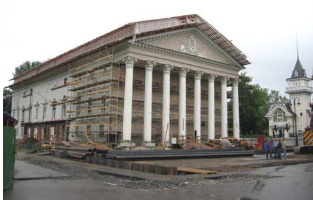
Figure 1. General view of the theatre during reconstruction
