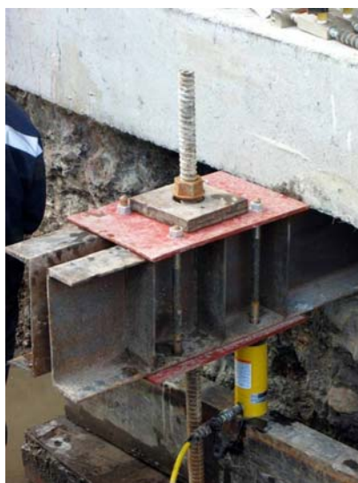
Figure 5. Underpinning piles support the whole structure
