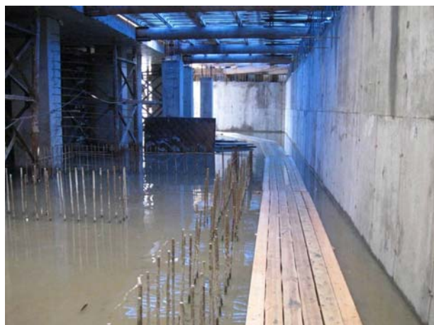
Figure 2. Construction of the underground part of the theatre
