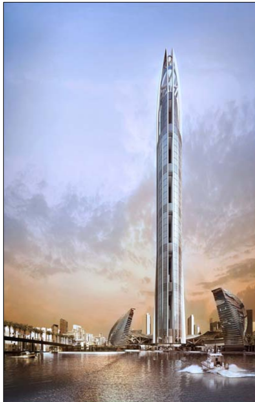
Figure 1: Nakheel Tower, Dubai, UAE
