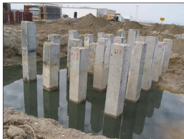
Figure 8. Driven piles at the location of approaching bridge pier
