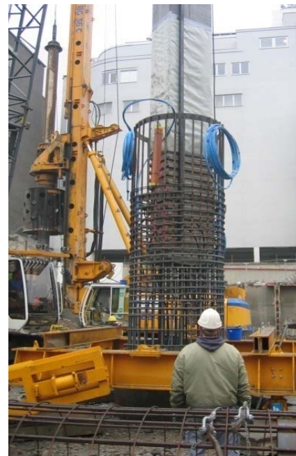
Installation of Energy Pile
