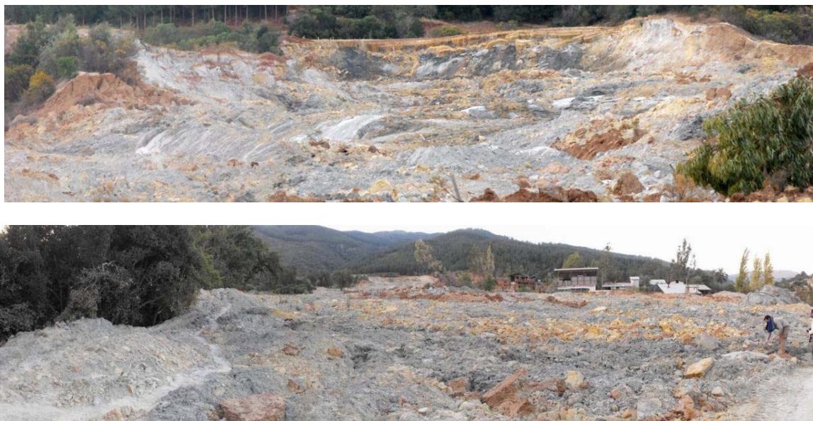
Fig. 7.- Mass of tailings remaining after flow failure
