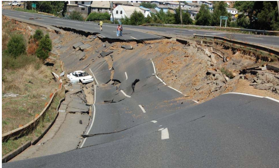
Fig. 5.- Failure of a fill triggered by foundation failure, Sector Polvorín, Ruta P160
