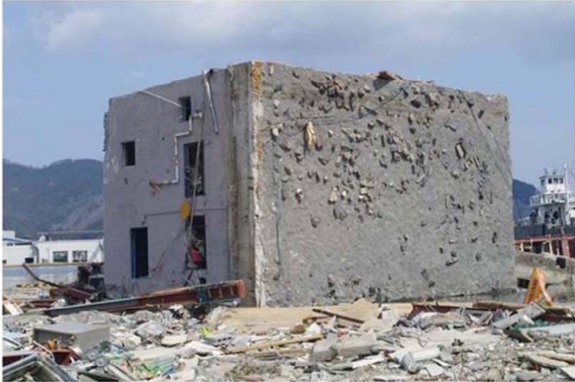
Overturned RC-building with shallow foundation. (Motoki Kazama, Tohoku University from Japanese Geotechnical Society (JGS) website : first results of its activities after the occurrence of the 11th March, 2011 Tohoku earthquake, http://www.jiban.or.jp/e/disaster-survey-information-of-2011-tohoku-earthquake-2/ )
