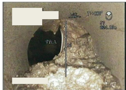
Photo 2. Disconnection of sewage pipeline and deposit of sand after liquefaction (damage study in Tokyo Bay area, 2011)
