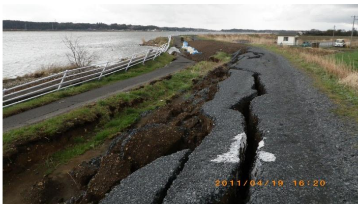
Photo 1. Liquefaction damage in Hinuma levee
