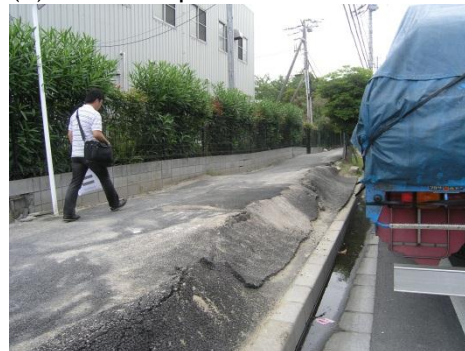
(b) Detail of uplifted sidewalk
