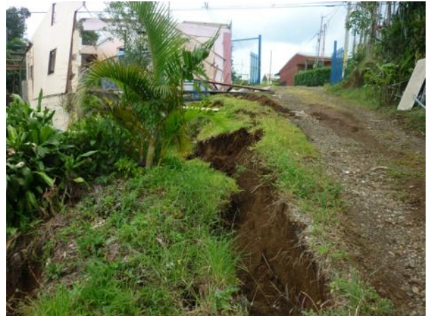
Fig. 15 Failure of unstable fill in Sarchi (Photograph by W. Vargas).
