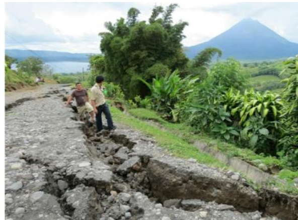
Fig. 16 Tension cracks and failure of a fill in La Fortuna (Source: La Nacion, online version).
