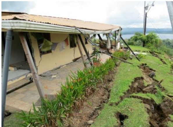
Fig. 16 Tension cracks and failure of a fill in La Fortuna (Source: La Nacion, online version).
