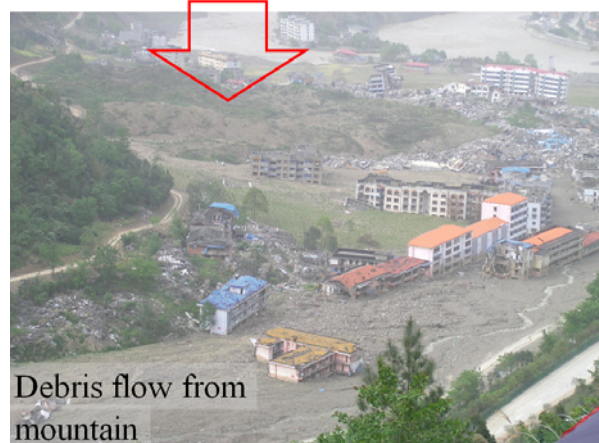
Fig. 6 Continued slope disasters in Beichuan after the earthquake on May 12th, 2008 (photograph taken on April 20th, 2009).
