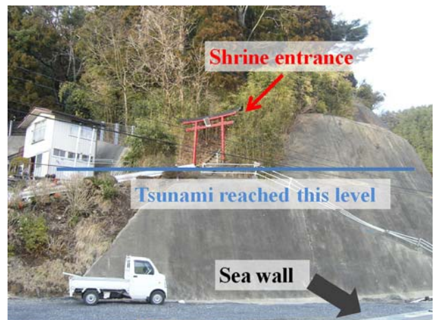
Fig. 24 Tsunami water level well above the sea wall and close to the entrance gate of a local shrine.
