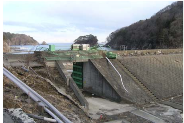
Fig. 22 High sea wall against tsunami attack (Karani-Hongo).
