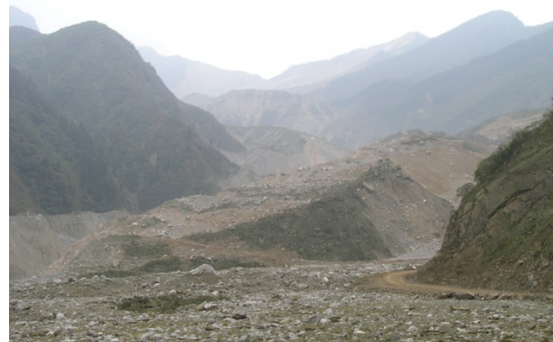
Fig. 9 Huge volume of debris deposits in the valley bottom at Wenjiagou.
