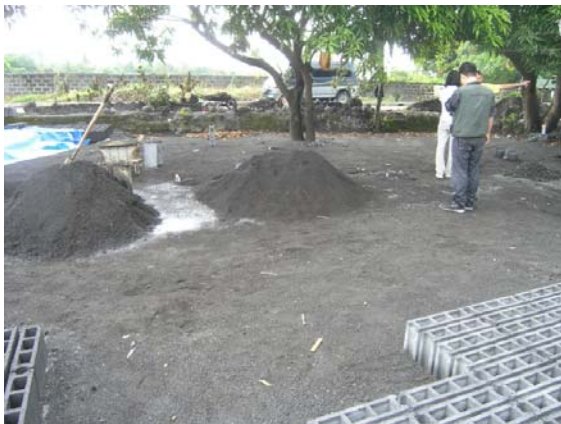
Fig. 17 Block production in lahar-prone village of Bunot.
