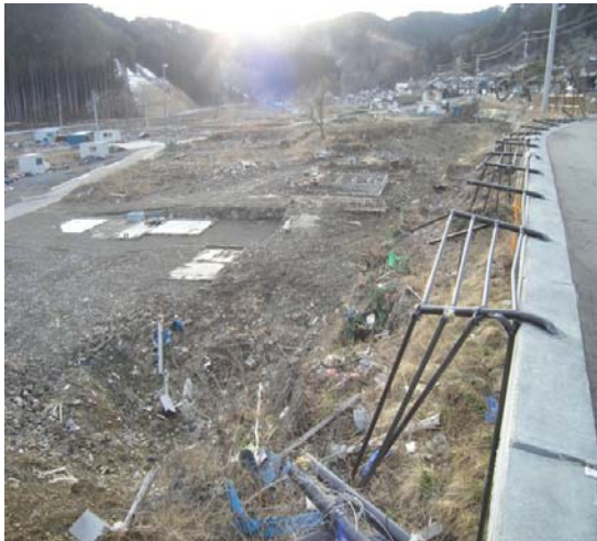
Fig. 23 Tsunami disaster behind the sea wall of Karani-Hongo (houses at higher elevations in the top right survived the tsunami).
