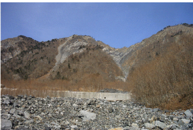
Fig. 3 Unstable Ohya slope.
