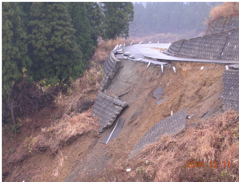
Fig. 22 Retaining wall sliding down with road embankment.
