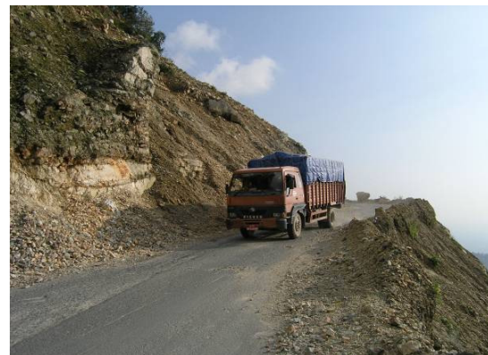
Fig. 6 Failure of cut slope at Sorchen.
