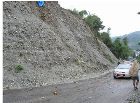
Fig. 13 Seismic falling of debris from cliff of terrace deposit in Phuntsholing.
