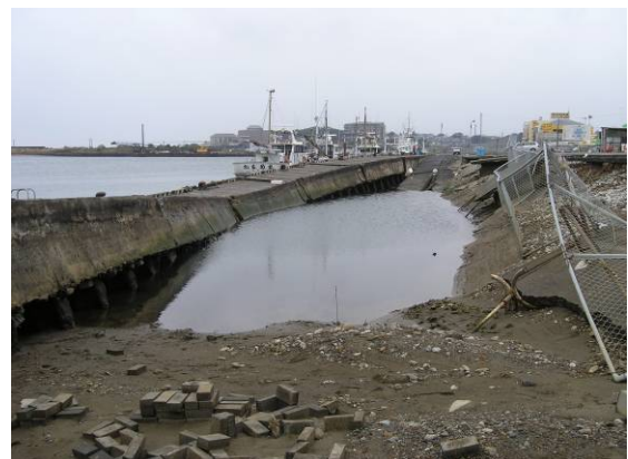
Fig. 20 Damaged quay wall in Nakaminato Harbor
