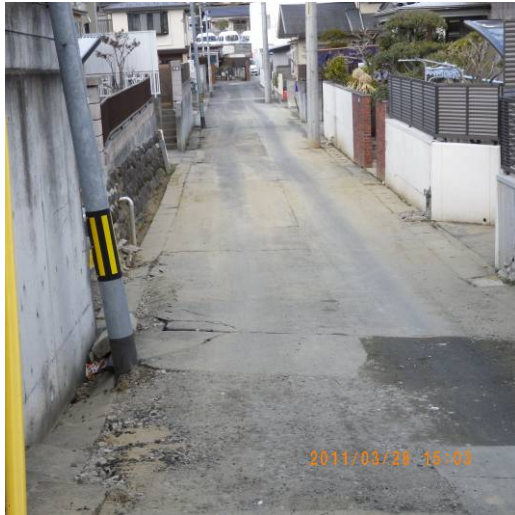
Fig. 38 Soil liquefaction in Asahigaoka 2 of Sendai City
