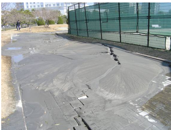
Fig. 14 Liquefaction in Urayasu City of Chiba
