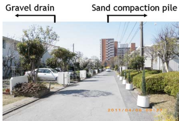
Fig. 30 Successful soil improvement in Irifune-Kita area of Urayasu residential area
