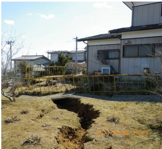
Fig. 36 Failure of residential development slope in Midorigaoka of Sendai City
