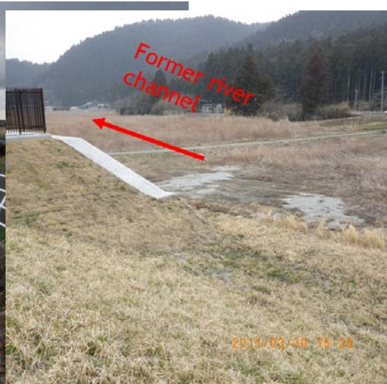
Fig. 28 Repeated liquefaction behind Eai River levee at Kita Wabuchi site
