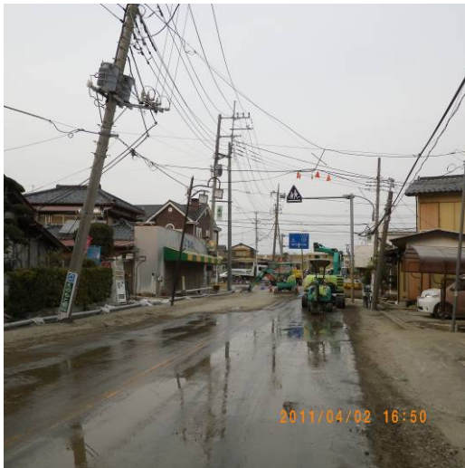
Fig. 23 Liquefaction in residential area of Abiko City (Fusa area)
