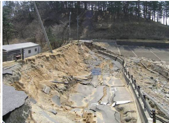
Fig. 41 Seismically breached Fujinuma Dam
