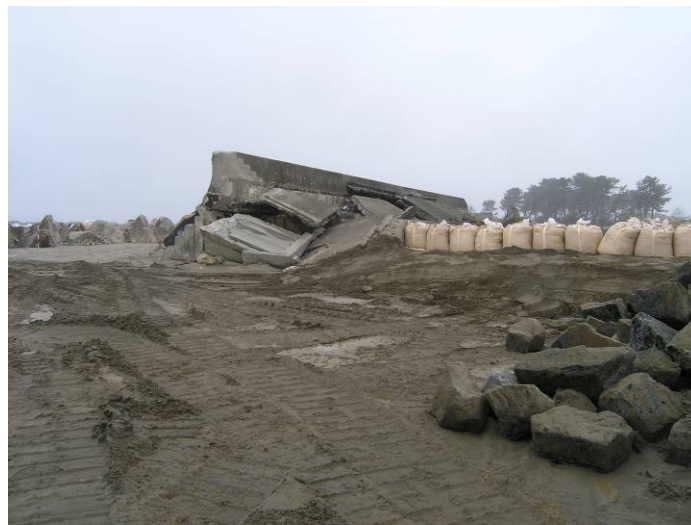
Fig. 13 Destroyed sea wall near Abukuma River mouth
