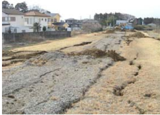
Fig. 25 Liquefaction-induced lateral spread of Naka River levee
