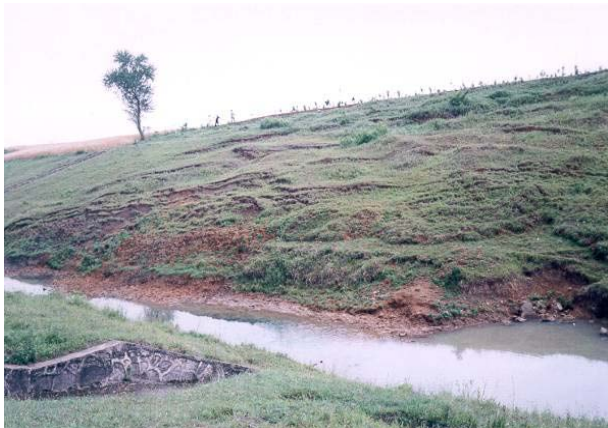
Figure 4 Typical shallow retrogressive failures at Dagangpo
