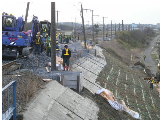
Fig. 34 Distortion of railway embankment (Joban Line of Japanese Railway East, near Mito, Ibaraki)
