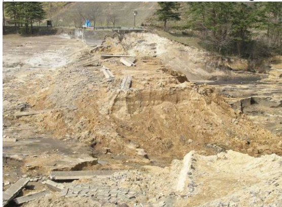
Fig. 41 Seismically breached Fujinuma Dam
