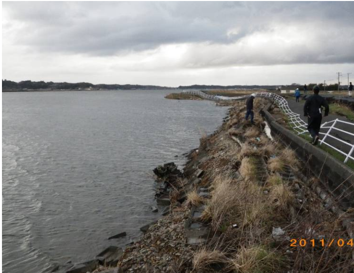
Fig. 27 Flattened Levee of Hinuma Lake near Mito City (Pechanko!)
