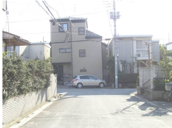
Fig. 17 Tilting of house (Mihama of Chiba)
