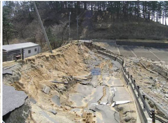
Fig. 41 Seismically breached Fujinuma Dam
