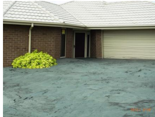
Figure 15. Damage to residential houses due to repeated liquefaction in Seabreeze Close, Bexley.
