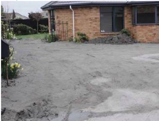
Figure 15. Damage to residential houses due to repeated liquefaction in Seabreeze Close, Bexley.
