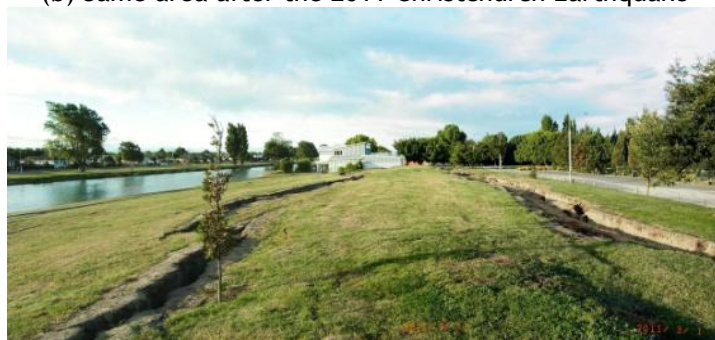
Figure 13. Lateral spreading and the crown settlement of a stop bank near Porritt Park.
