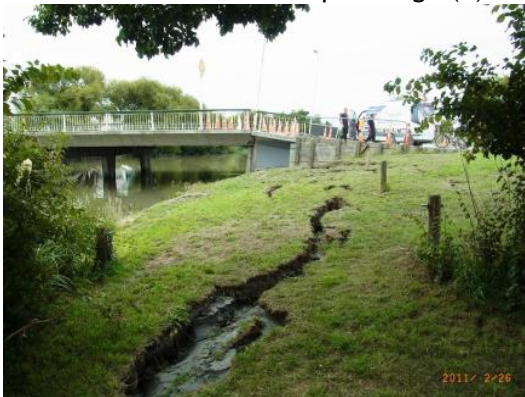
Figure 16. Damage to bridge crossing the Avon River (Avondale Road).
