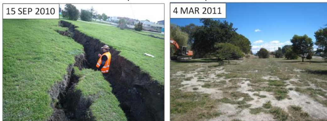
Figure 21. Damage to the stop bank along Kaiapoi river (North Kaiapoi). Sand boils were observed on restored cracks. The damage to the stop bank was minor and lots of small fissures were observed at restored cracks.
