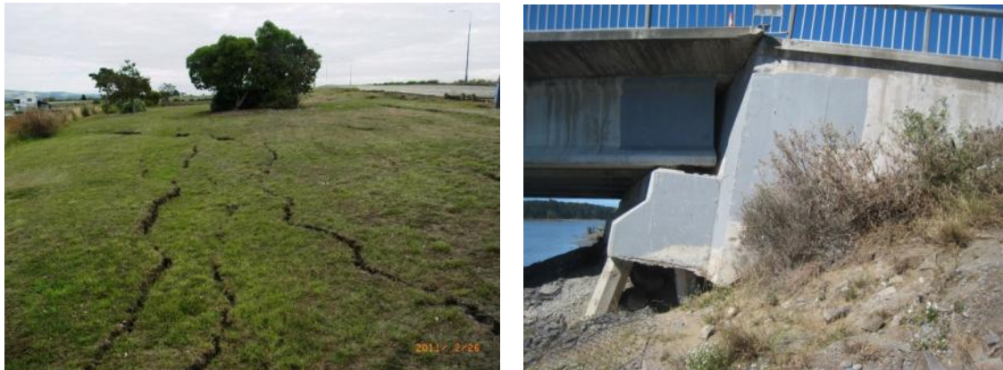
Figure 18. Liquefaction-induced damage to South Brighton Bridge.
