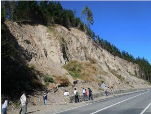
Failure of coastal slope near Concepcion
