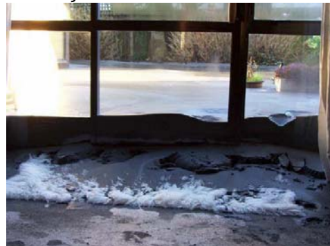
(c) View from the street (before clean up); (d) liquefied silt-sand-water mixture covering a rug inside the house and the ground outside the house (seen through a window from inside the house)
