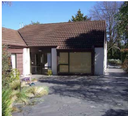
(a) ~40 cm thick layer of silt-sand-water mixture covering a residential property affected by very severe liquefaction; (b) same-angle view, but after the clean up of sand ejecta
