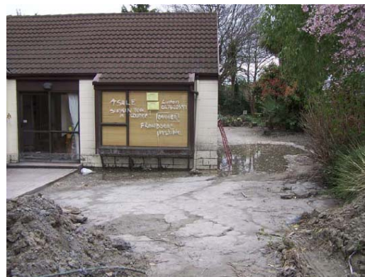
(a) ~40 cm thick layer of silt-sand-water mixture covering a residential property affected by very severe liquefaction; (b) same-angle view, but after the clean up of sand ejecta
