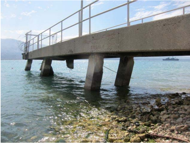
Figure 9 Damage to piles supporting the pedestrian bridge connecting the South Pier to the island
