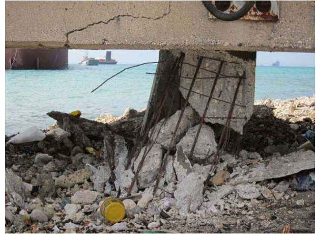
Figure 9 Damage to piles supporting the pedestrian bridge connecting the South Pier to the island
