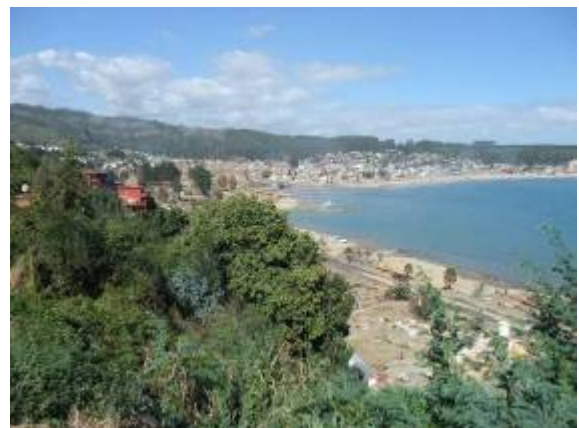
Photo 22 Tsunami erosion in coastal area of Dichato
