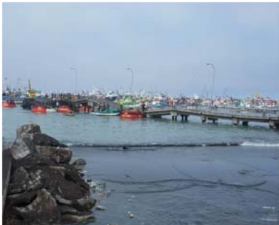
Photo 18 Damaged pier in Coronel
