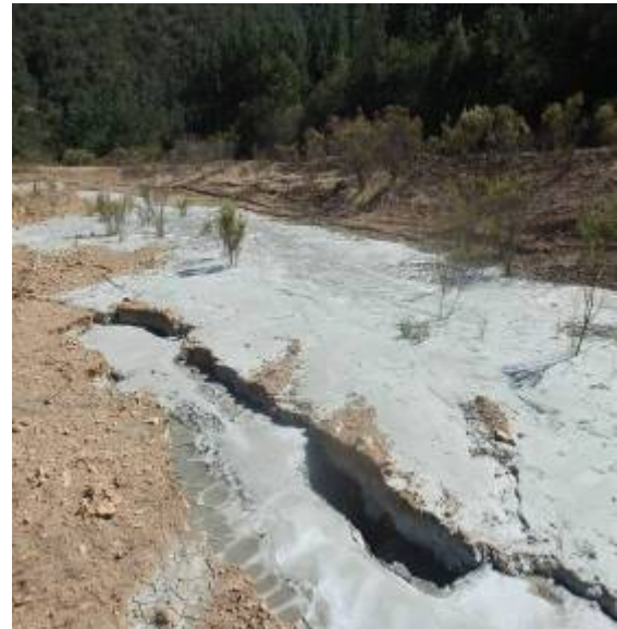
Photo 8 Eruption of liquefied tailings at Las Palmas
