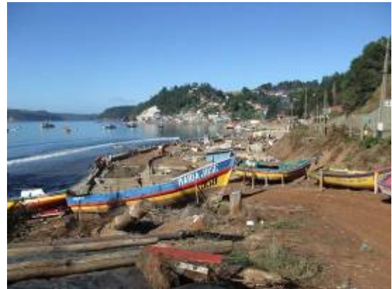
Photo 20 Tsunami damage near Cape Blanca
