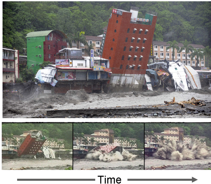
Figure 29. Erosion-induced failure of river wall and collapse of building
