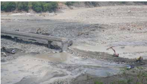
Figure 19. Bridge abutment and embankment destroyed by erosion
