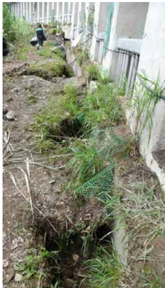
Figure 16. Subsidence in foundation of rock-shed tunnel
