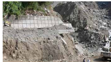
Figure 9. Collapse of retaining wall without stable foundation
