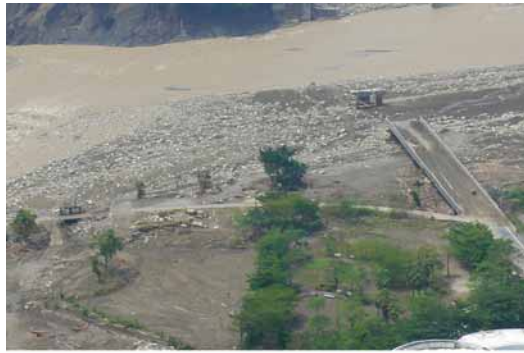
Figure 18. Destroyed bridge because of scouring
