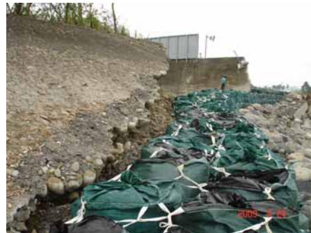
Figure 20. Erosion at toe of road embankment
