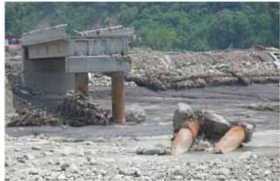
Figure 35. Scouring in bridge foundation
