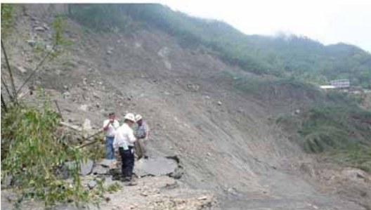
Figure 13. Mountain road destroyed by slope failure
