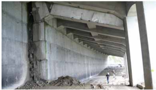
Figure 15. Distortion of rock-shed tunnel
