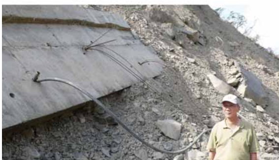
Figure 10. Destroyed shape of ground anchor.
