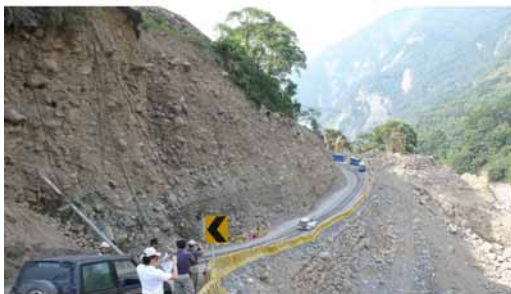
Figure 8. Failure of natural slope along road
