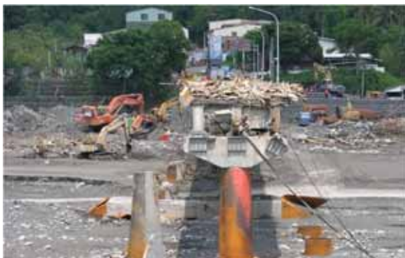
Figure 36. Accumulation of drifting wood on bridge deck
