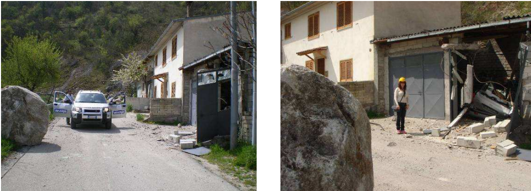
Figure 9. Rockfall at Fossa: the rock fell from the hill on the right, crossed the garage and stopped across the street.
