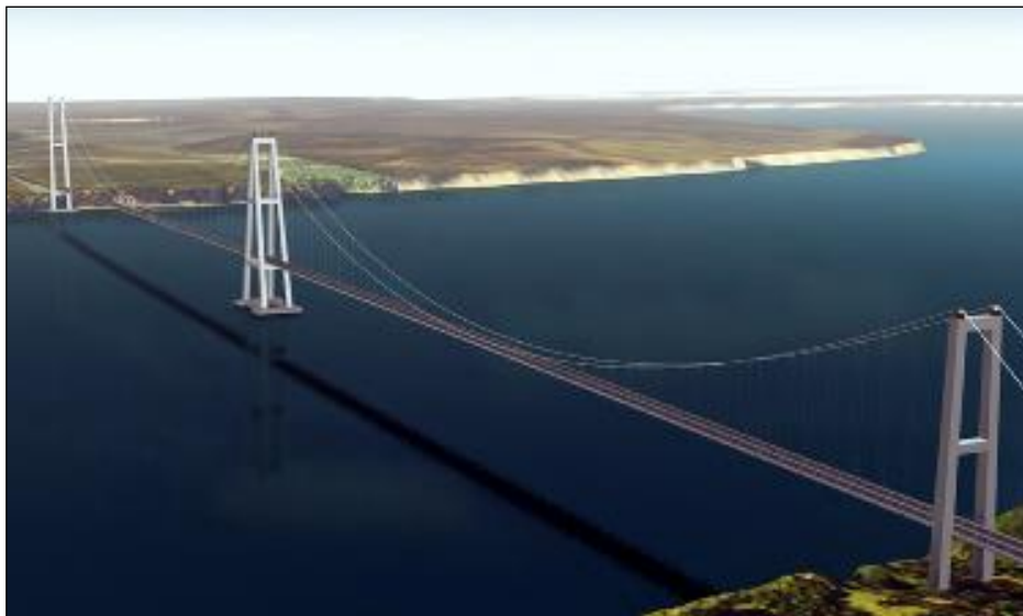
Figure 1. The project consider the construction of about 2.5 km long double suspension bridge, been after its construction, the largest suspension bridge in South America
