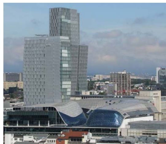
Figure 7 Project "PalaisQuartier", Frankfurt am Main, Germany
