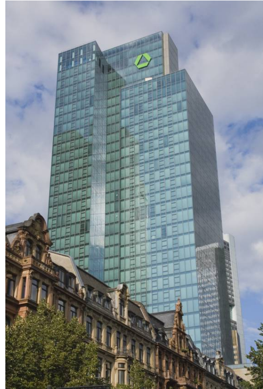
Figure 22 View on the finalised high-rise building
