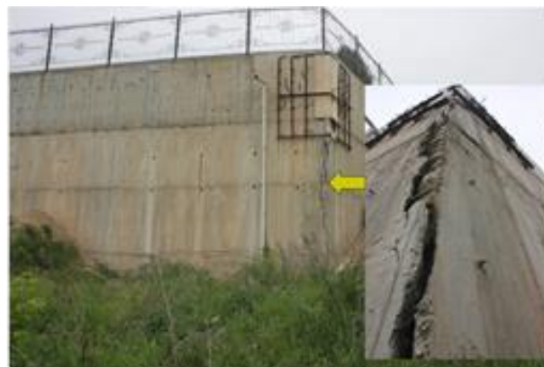
Fig. 2. Opening cracks in the corners of the retaining wall.
