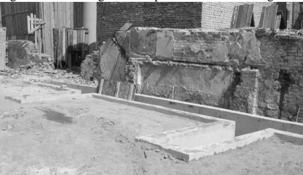
Fig. 4. Constructed guiding walls with counterforts
