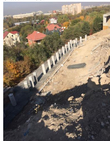
Fig. 5. General view of the reinforcement of the retaining wall after the installation of bored piles.
