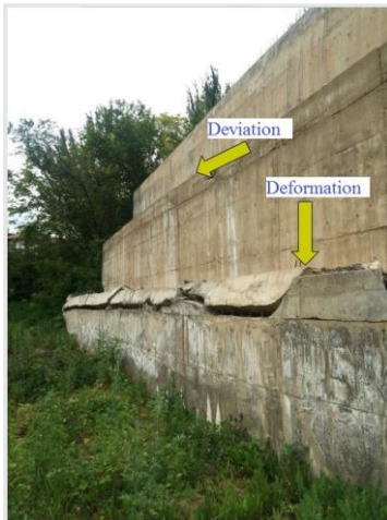
Fig. 6. Deformation and destruction of concrete retaining walls.
