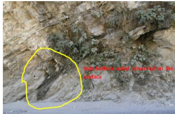
Fig. 9. Water seeping through jointed rock-mass
