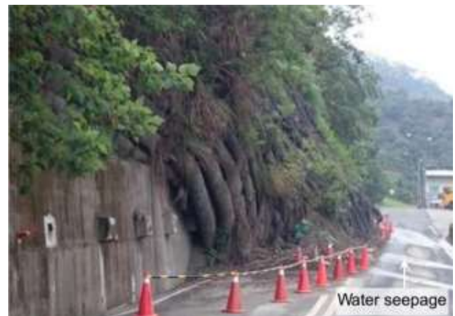
Figure 2. A GRS structure failure triggered by rainfall
