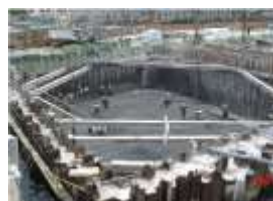
(2) Excavation and assembling steel bar of river slab
