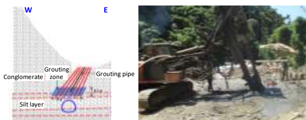
Fig. 12. Ground improvement grouting in earth surface.
