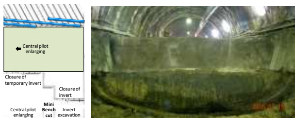
Fig. 11. Mini bench cut and closure of invert.
