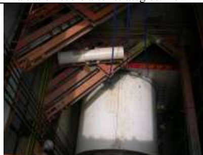
Figure. 5. The proceeding of shield machine.
