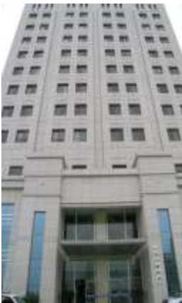
(a) A 12-storey frame-shear wall building on a Loess Yuan with about 200m loess deposit.
