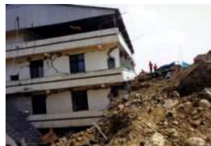
Fig. 1. Damages of building caused by reverse faulting in the 1999 Chi-Chi earthquake (Provided by W.J. Huang, NCU)
