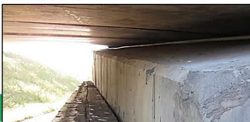
Figure 3. Cracking and spalling of corners of RF panels on main south abutment wall.
