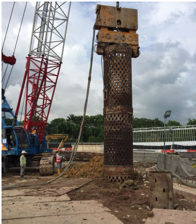
Fig. 9. Perforated steel casing used as a pressure relief system
