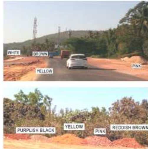
Fig. 4. Photo showing the usage of different colored lateritic soils in embankments in Goa
