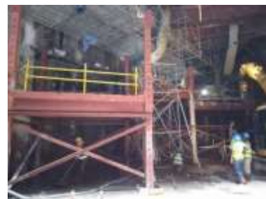
(a) Working lift fabricated in vertical shafts
