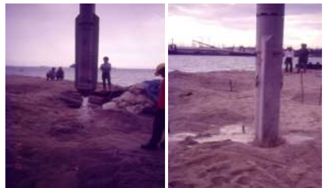
Fig. 15. Only bottom jets available – no annular space created
