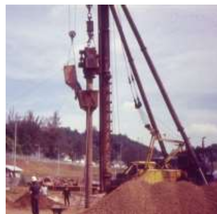
Fig. 21. Step by step feeding – conventional execution
