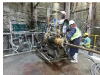
(b) Execution of horizontal jet grouting
