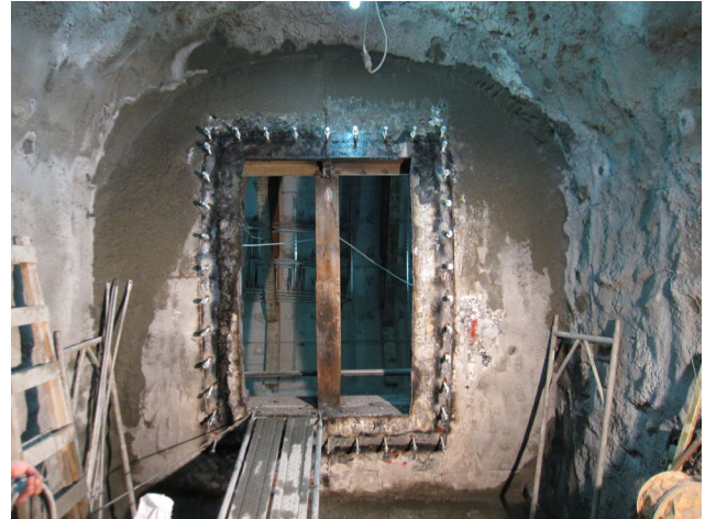
Fig. 6. The steel segments removal.
