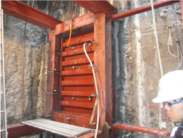
Fig. 4. The safety gate at the shaft side.
