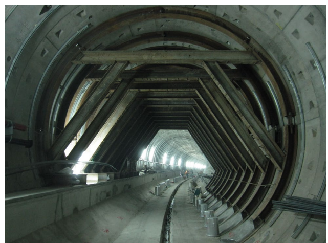
Fig. 3. Steel rings of protecting tunnel segments.
