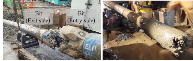
Fig. 10. Intersection construction and bit balling photo
