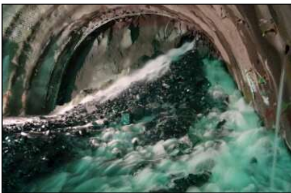
Fig. 5 Eruptive massive inflow at station of 7K+200.5
