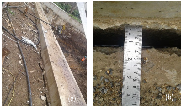
Fig. 4 (a) Gap between the wall and the soil @ 30mm wall movement (b) @ 45mm wall movement after rains
