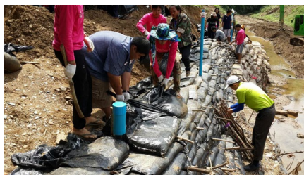
Fig. 4. Placement of flapped soil bag with live stake
