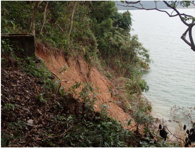
Fig. 5. Coastal slope possibly experienced an upward extension of failure following the loss of toe mass due to erosion.
