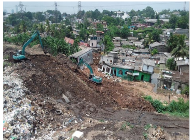
Fig. 1. Damage due to the failure of the garbage fill
