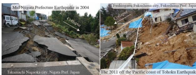
Fig. 7 Collapse of the fill slope from the embankment slope
