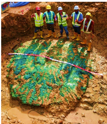
Fig. 8. Exposed Jet Grouting column of T01 with a diameter of 3.5 m.
