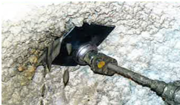
Fig. 1. Overflowing mortar out of a rock bolt hole on tunnel crown.
