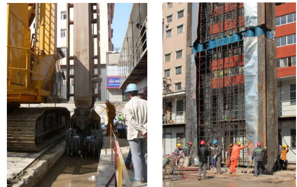
Fig. 8 The excavation and lowering of the steel cage (loadcell)
