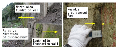
Photo. 5. Residual horizontal displacement toward mountain side induced by intense ground motion
