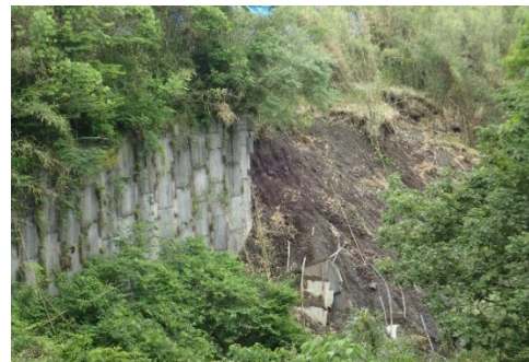
Photo. 1. Adjacent failed and remaining reinforced soil wall
