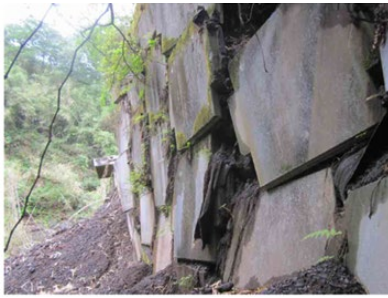
Photo.3. Self-standing facing of failed reinforced soil wall
