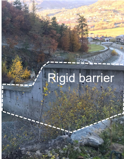
Fig. 1. Rigid barrier to resist debris flow
