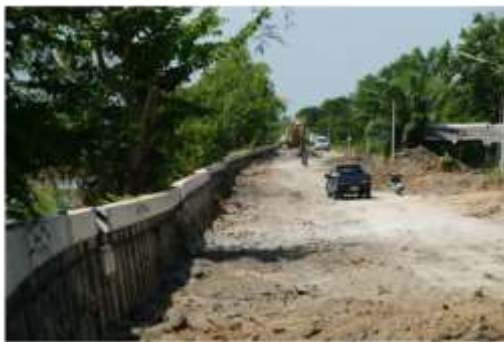
Figure 7 : Failure of embankment along Canal Bank
