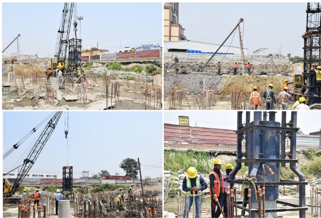
Fig. 7. Instrument brought to perform HSDT test at the Uttarakhand site in India
