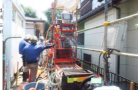
Figure 4 Ground improvement by jet grouting in a narrow space
