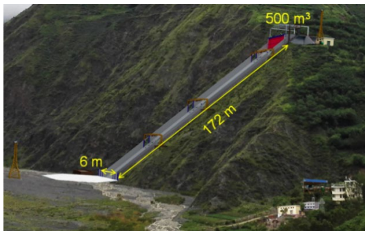
Fig. 15. Schematic of 172 m-long flume in Kunming, China
