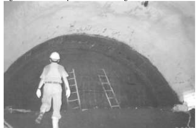
Fig. 7. Excavation of top-heading.
