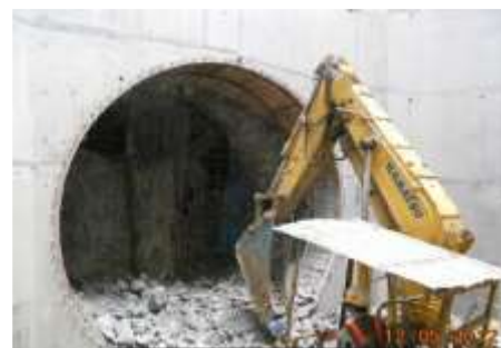
Fig. 11. Demolish work of #2 shaft.
