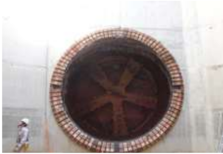
Fig. 13. Install watertight ring of tunnel face.
