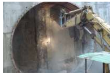
Fig. 10. Demolish the wall of #2 shaft.
