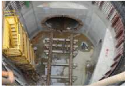
Fig. 14. Set up the arrival platform of shield machine.
