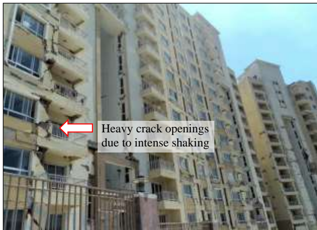
Fig. 1. A typical damage scenario of a 17-story apartment building (Location no. 22 in Fig. 2) on raft foundation in the Kathmandu Valley.
