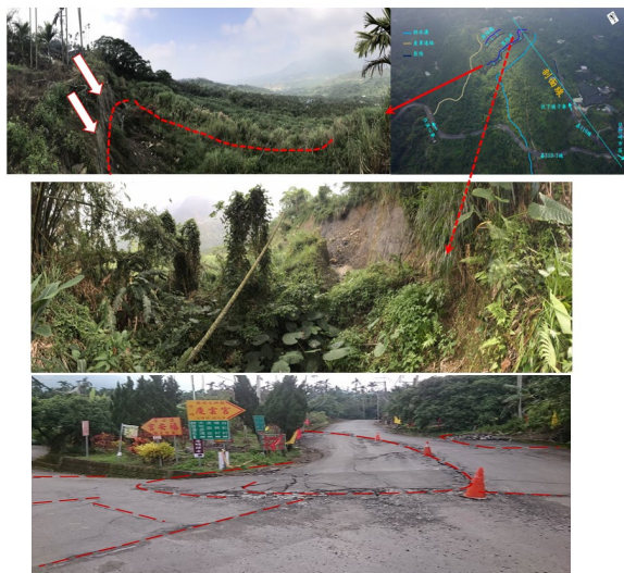
Fig. 11. Head scarp at top of slope and cracks in the national route No.119
