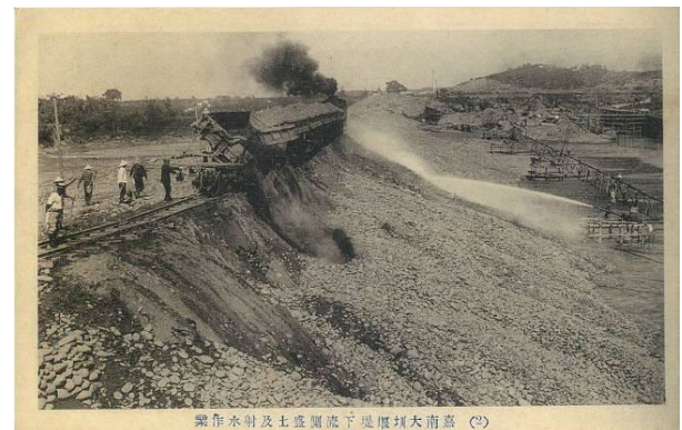
Fig. 7. Earth material discharge and water injections.
