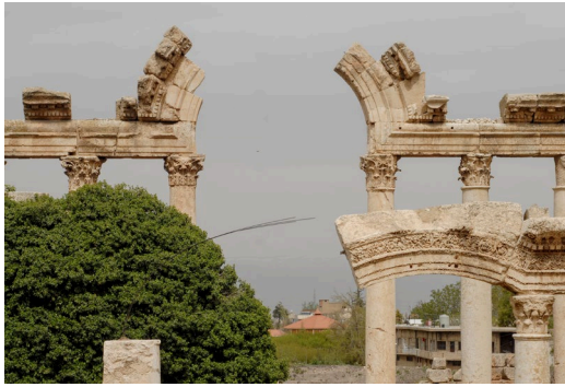
Fig. 4: Bustan el-Khan, Baalbek (Lebanon). Post-tensioning intervention of Kalayan. See Miller (1971) for technical details and comments: "Structural tricks of cantilevered architraves and arches can defy gravity in deference to aesthetic judgement". Photo: P. Smars, 2015
