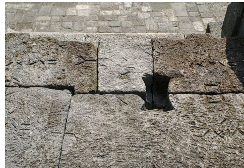
Fig. 8: Borobudur (9th c. CE), Indonesia. Dovetail socket, assembly marks and indented joints. Photo: P. Smars, 2014.
